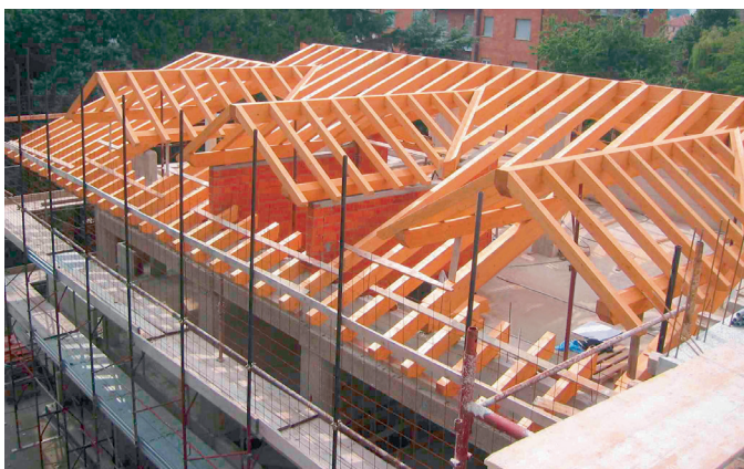
Production of roof structures directly from CAD/CAM
