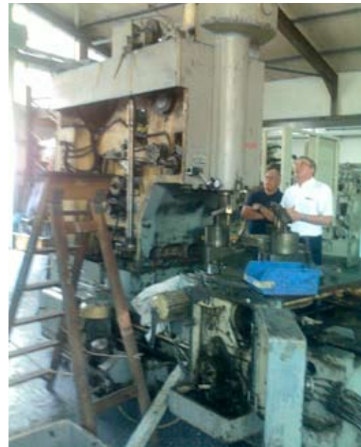
„Before“ – starting the rebuild
