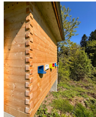
Appenzell-Style Joinery Featured Throughout the Apiary – Inside and Out
